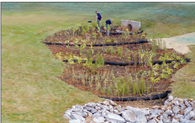
Figure 7–4. A grassed channel leading from a partially visible strip mall (A) before and (B) after construction of a stormwater management channel leading to an outfall pipe in Lynchburg, Va. The previously grassed channel was converted to a wetland to reduce runoff and filter pollutants. (Photographs by Center for Watershed Protection, Ellicott City, Md.)
