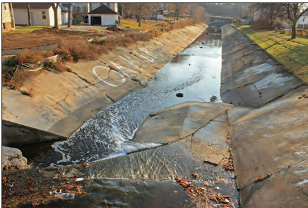
Figure 7–2. Habitat is being restored along the Kinnickinnic River in Milwaukee, Wis., to improve fish passage and reconnect the stream to the flood plain.
