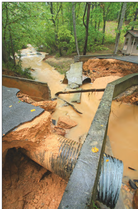
Figure 1–2. Frequent high flows increase the potential and severity of erosion, habitat degradation, and destruction of road crossings and infrastructure. This road crossing was washed out during a flood near Atlanta, Ga., in 2009.
