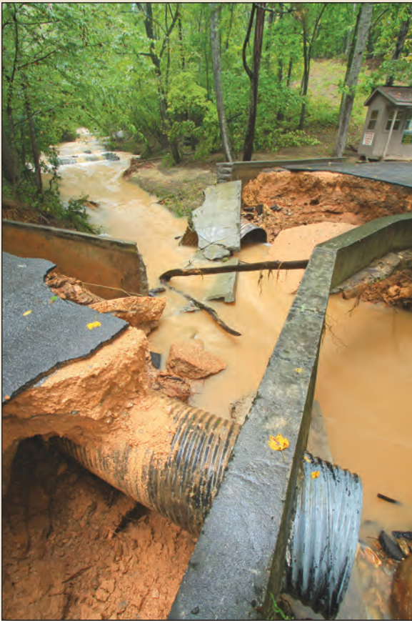
Figure 4–6. Frequent high flows increase the potential and severity of erosion, habitat degradation, and destruction of road crossings and infrastructure. This road crossing was washed out during a flood near Atlanta, Ga., in 2009.
