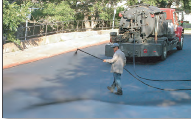
Applications of coal-tar-based sealcoat, applied to asphalt pavement, such as parking lots and driveways, can be a major source of PAH contamination in stormwater runoff. (Photograph from Van Metre and others, 2006.)
