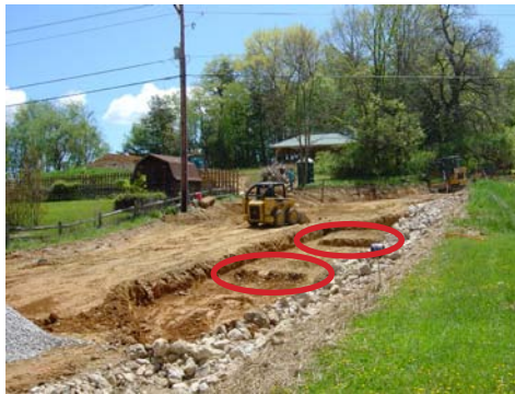
Figure 8. The top illustration shows a diversion mound system as used on a roadway. The photo to the left shows the installation of diversion mounds for an access road. The diversion mounds are circled in red. In the photo to the right you can see the mounds during the structural soil installation process.
