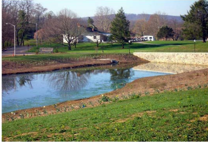
Figure 3. An example of a retention/detention pond adjacent to a conference center on the Virginia Tech campus in Blacksburg, Virginia. This treatment uses space that could be otherwise directed towards other uses.
