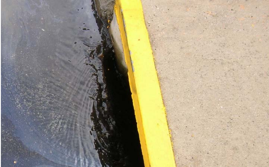
Figure 1. Typical runoff from a parking lot going into a storm sewer. Notice that traces of oil are visible to the naked eye. There are many other pollutants in parking lot runoff such as various metals, sediment, salts, and litter.
