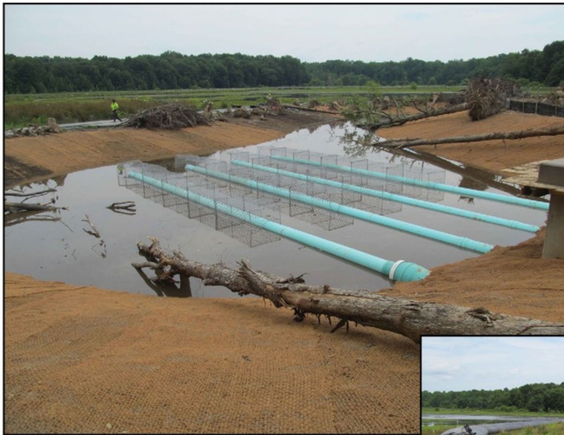
Clemson Water Levelers. Inset: Aqua-Dam in place.
