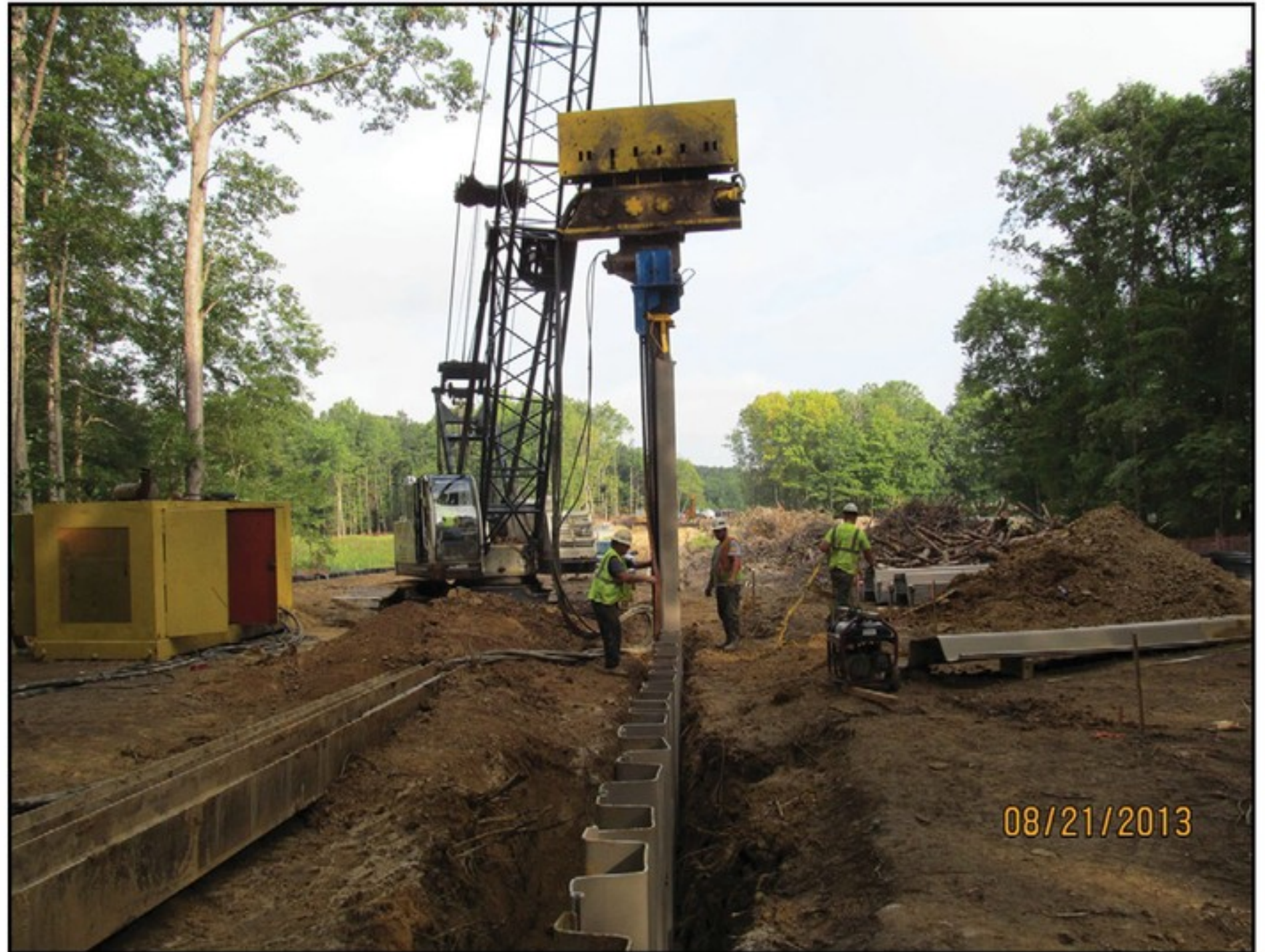
Sheet pile installation of water control berm.
