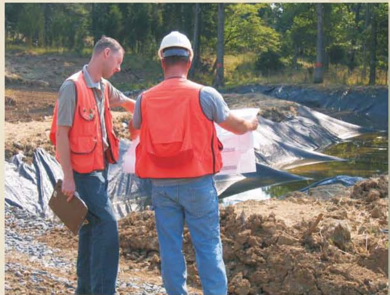
On-Site Sediment Control Inspections
