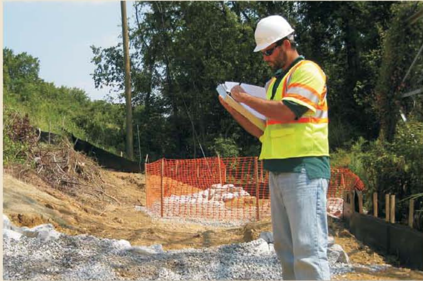
VSMP Site Inspection - Tysons Corner, VA
