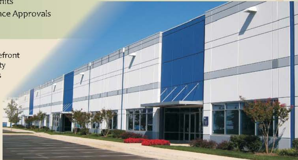
Beaumeade Corporate Park; Wetland Delineation, Survey, and Permitting - Ashburn, VA
