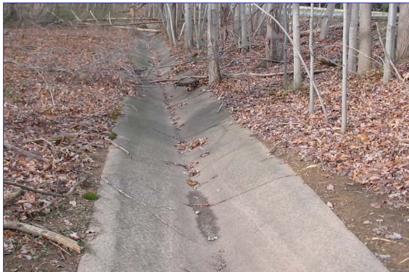
OPTION 2: Open Channel lined with concrete
