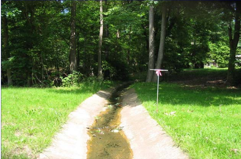
RCI = 0.25: Urban/suburban stream in Northern Virginia. Man-made, concrete channel.
