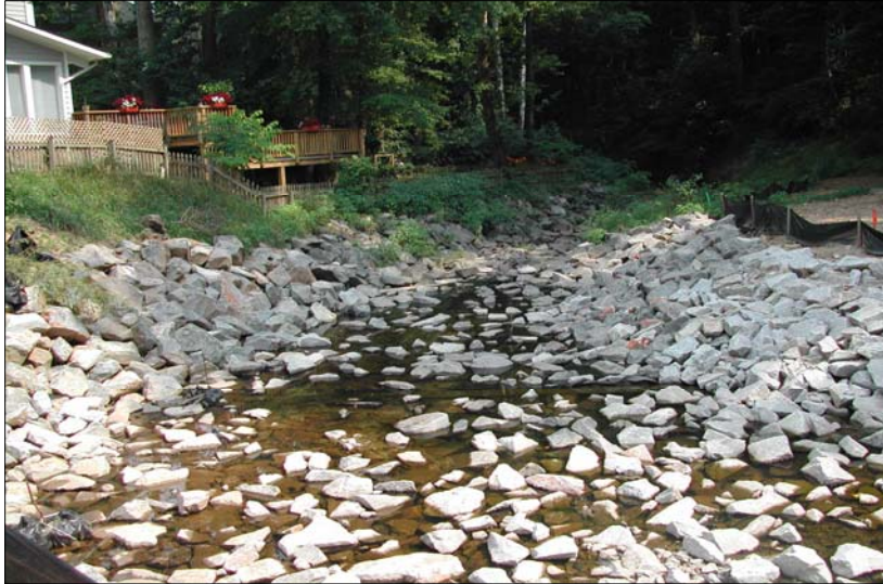
RCI = 0.50: Urban/suburban stream in Northern Virginia. Man-made, riprap channel.
