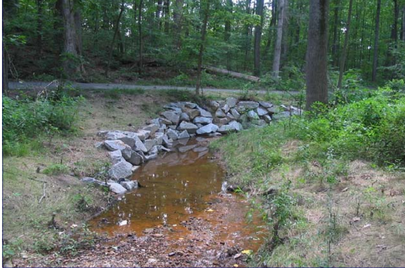
RCI = 3.8: Urban/suburban stream in Northern Virginia. Suboptimal channel condition; suboptimal riparian corridor; marginal in-stream habitat; fair benthos; moderate channel alteration.
